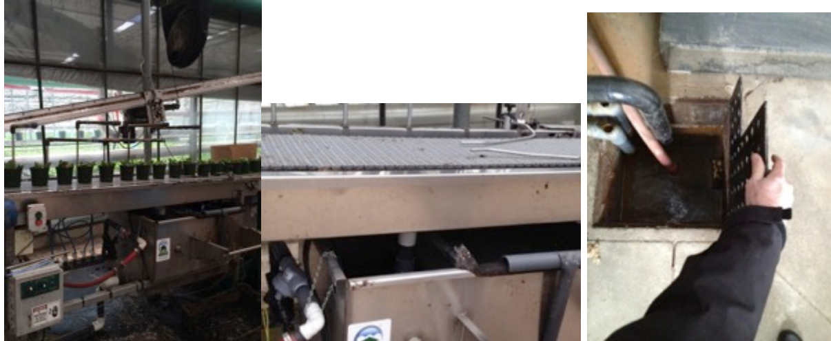
Figure 6. Planting line and the undertray to collect the water, and a floor drain
