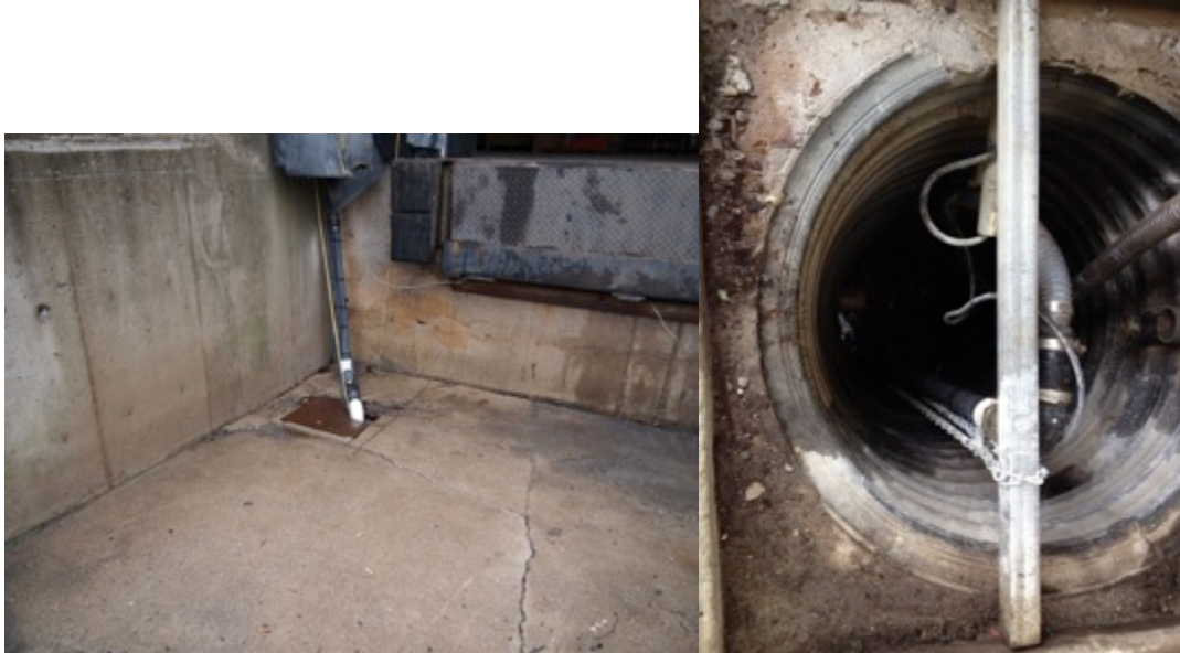
Figure 1. Loading dock (left), with the sump pit (right)
