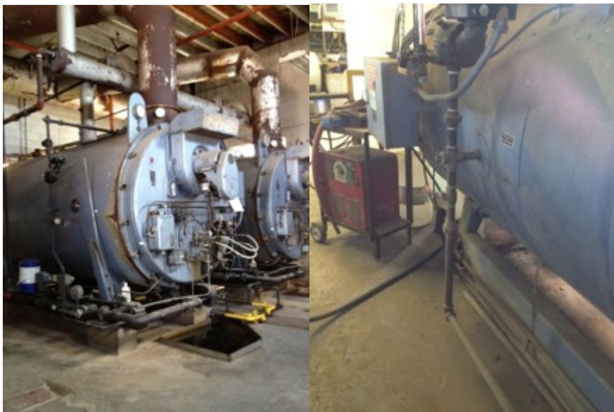
Figure 4. Steam boilers (left), with the blowdown access port (right)
