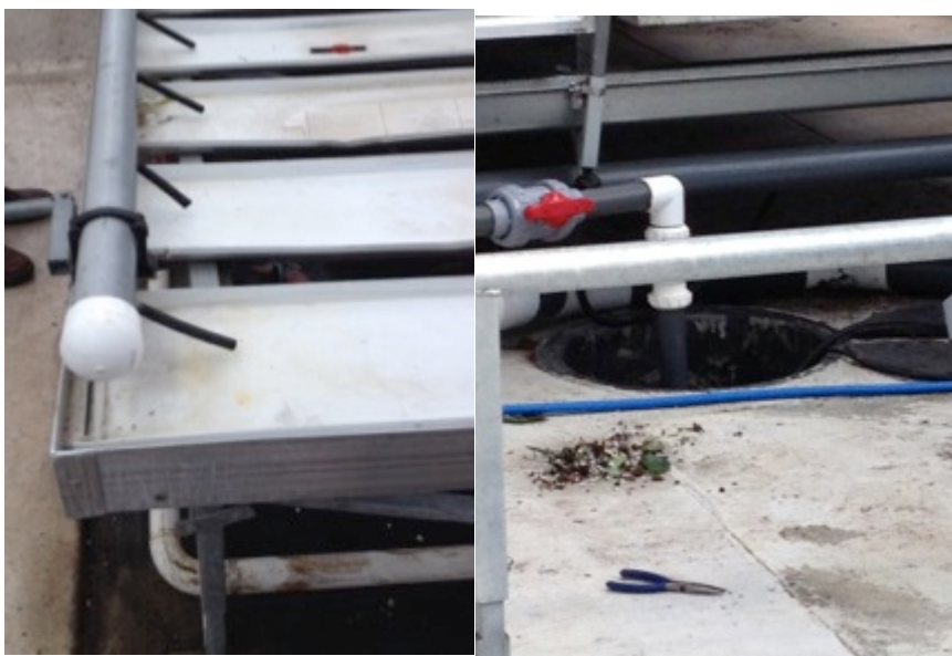
Figure 3. Under bench return tanks for recirculated nutrient feed water
