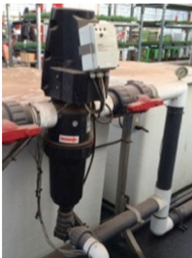
Figure 9. Filter near fertilizer feed tanks.
