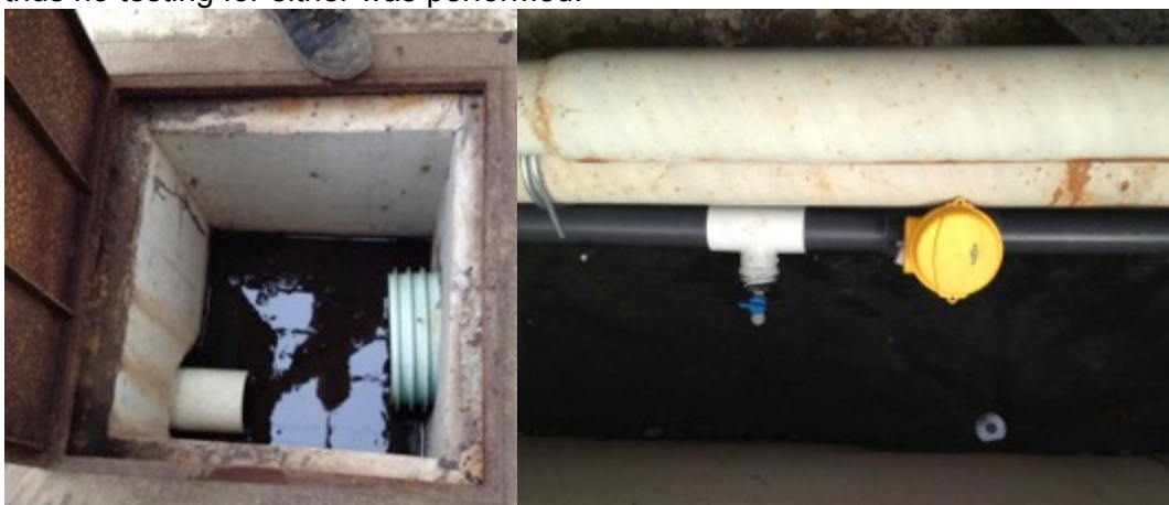
Figure 11. Isolating water streams in a catch basin (left), and installed flow magmeter (right)
