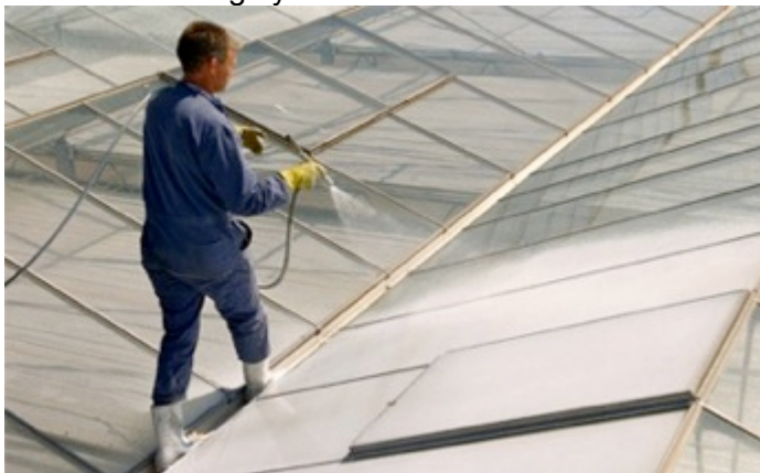
Figure 2. Applying whitewash
