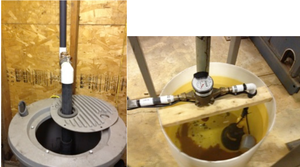
Figure 5. Boiler flue condensate collection, with sump pits and flow meters
